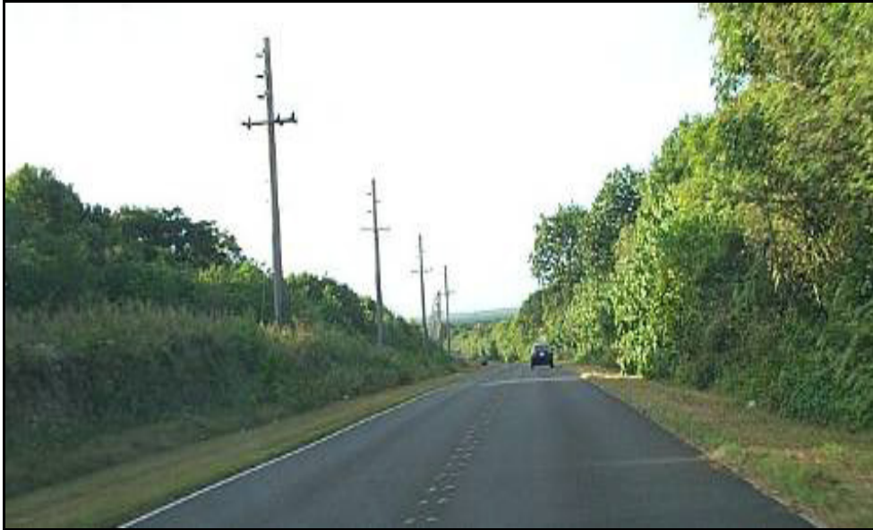
Figure 4.1-9. Typical Roadway Surface along Route 9
