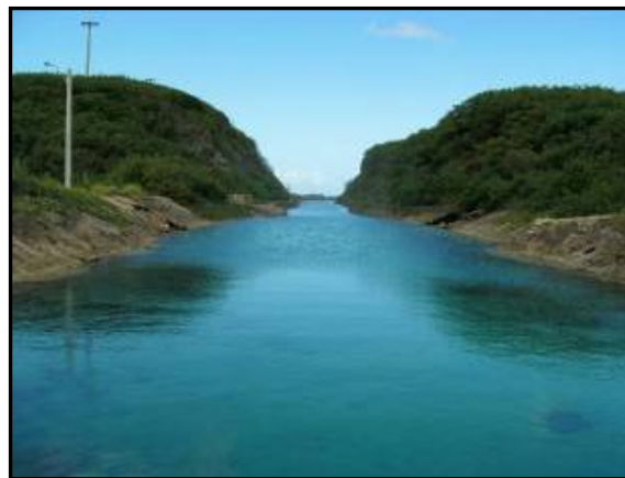
Right: Cooling water canal (Approximately 5 ac (2 ha) with rip rap lining the sides. This canal connects the power plant near the Commercial Port along Route 11 to Piti Bay and the Philippine Sea.
