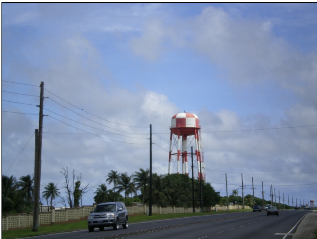
Figure 13.1-18. View from Route 3 Looking Northward with South Finegayan Water Tower in Foreground and NCTS Finegayan Water Tower in Background as Seen from Route 3 Looking North (Former FAA Parcel Lies in Between the Two)
