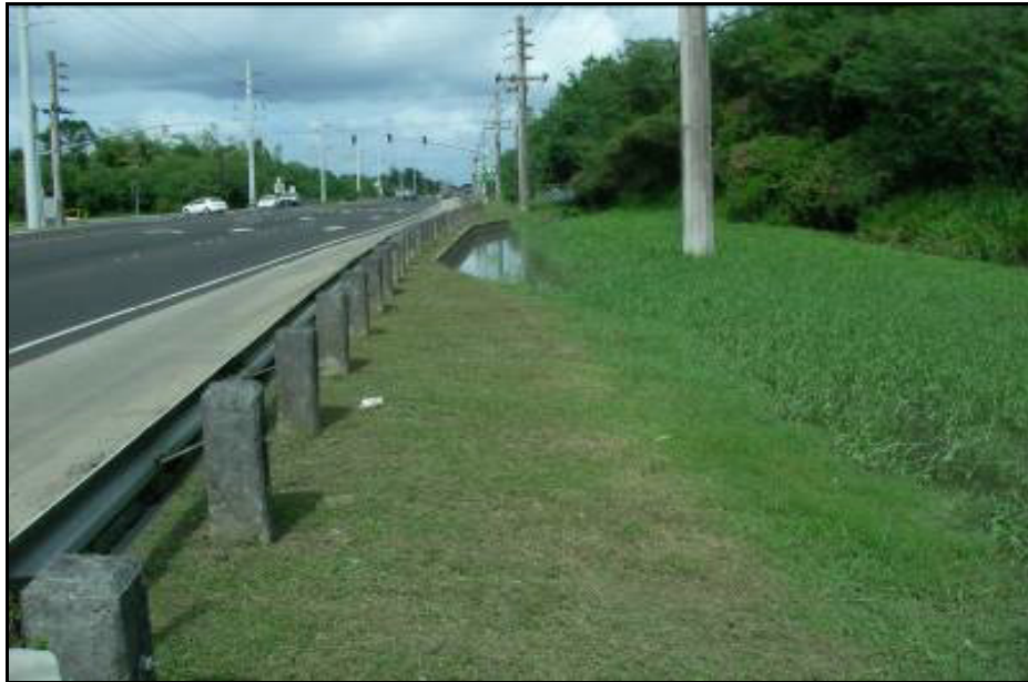
Figure 4.1-33. Route 1 at Laguas River Bridge
