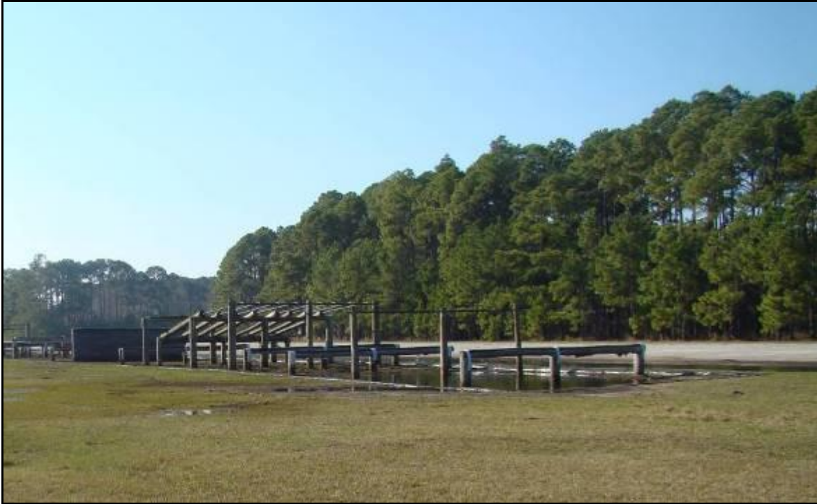
Figure 2.3-1. Typical Marine Corps Obstacle Course
