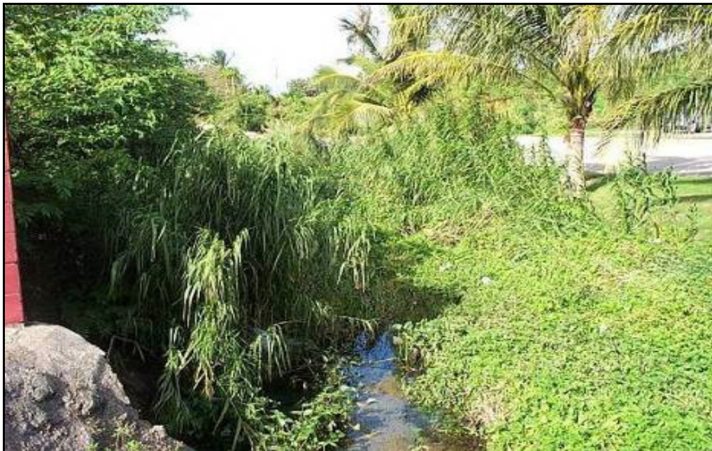
Figure 4.1-18. Tamuning Drainageway Downstream Channel
