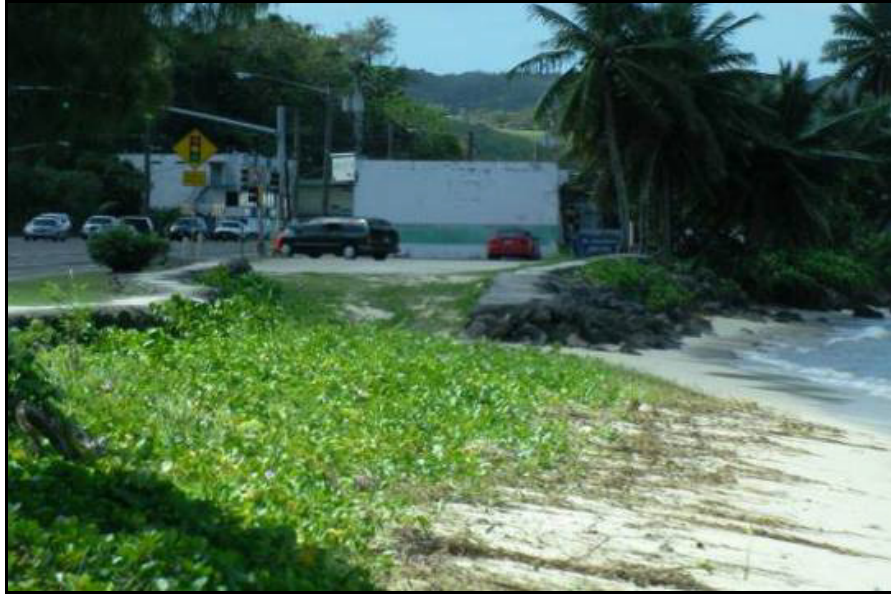
Figure 4.1-27. Coastal Erosion Protection along Route 1
