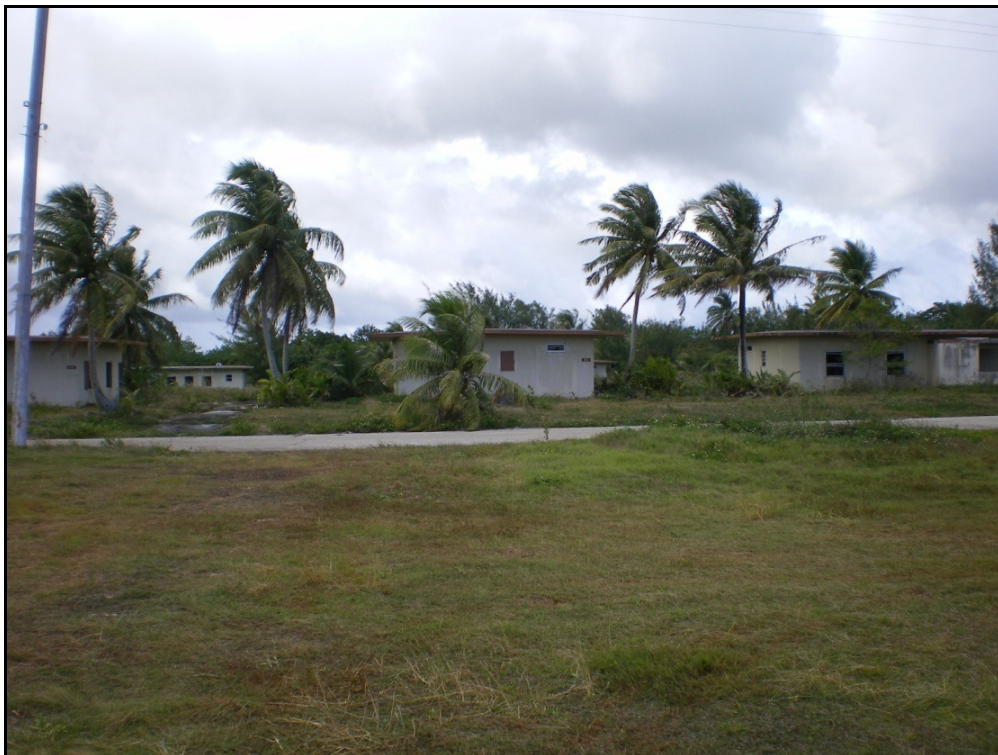
Figure 13.1-32. View of Abandoned Housing at Andersen South Source: EDAW 2009.
