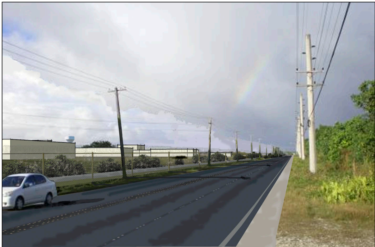
Figure 13.2-14. Alternative 3: View from Route 3 Looking Northward into the North Part of NCTS with New Facilities in the Foreground and Water Tower/Tank in the Background (RESULTING VIEW) Source: EDAW 2010.
