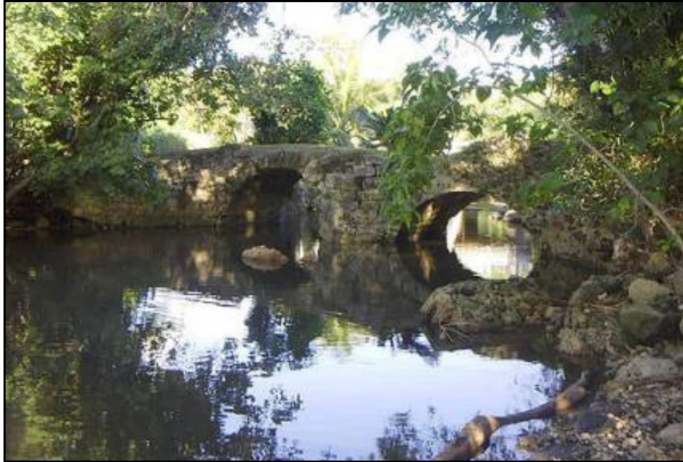
Figure 13.1-63. Talifak Spanish Bridge
