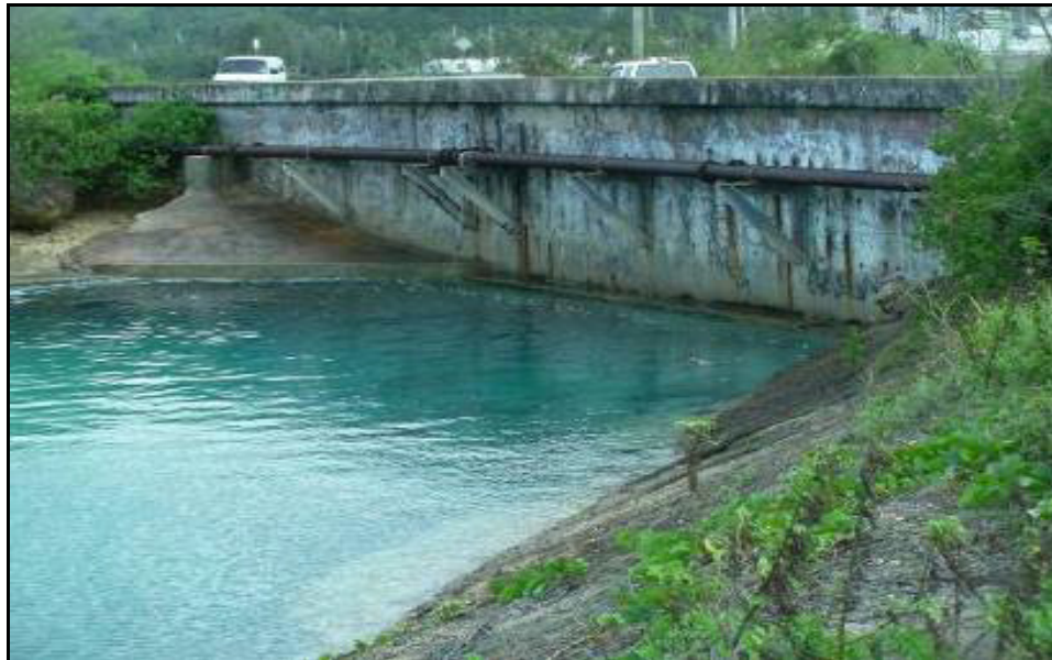
Figure 4.1-36. Route 11 Bridge over Piti Canal
