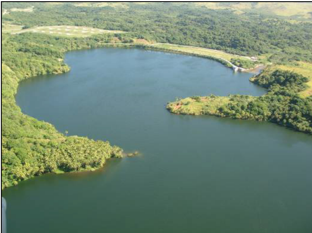
Figure 13.1-57. Fena Valley Reservoir
