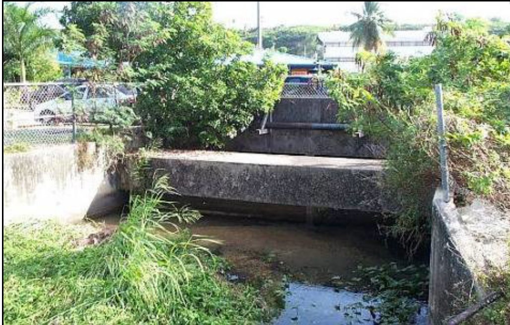
Figure 4.1-17. Tamuning Drainageway Outlet
