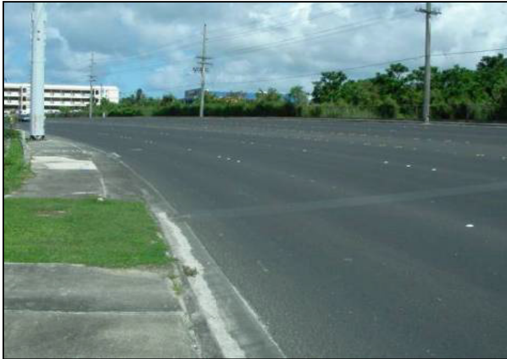
Figure 4.1-19. Route 16 – Curb Outlet at Low Point to Sink
