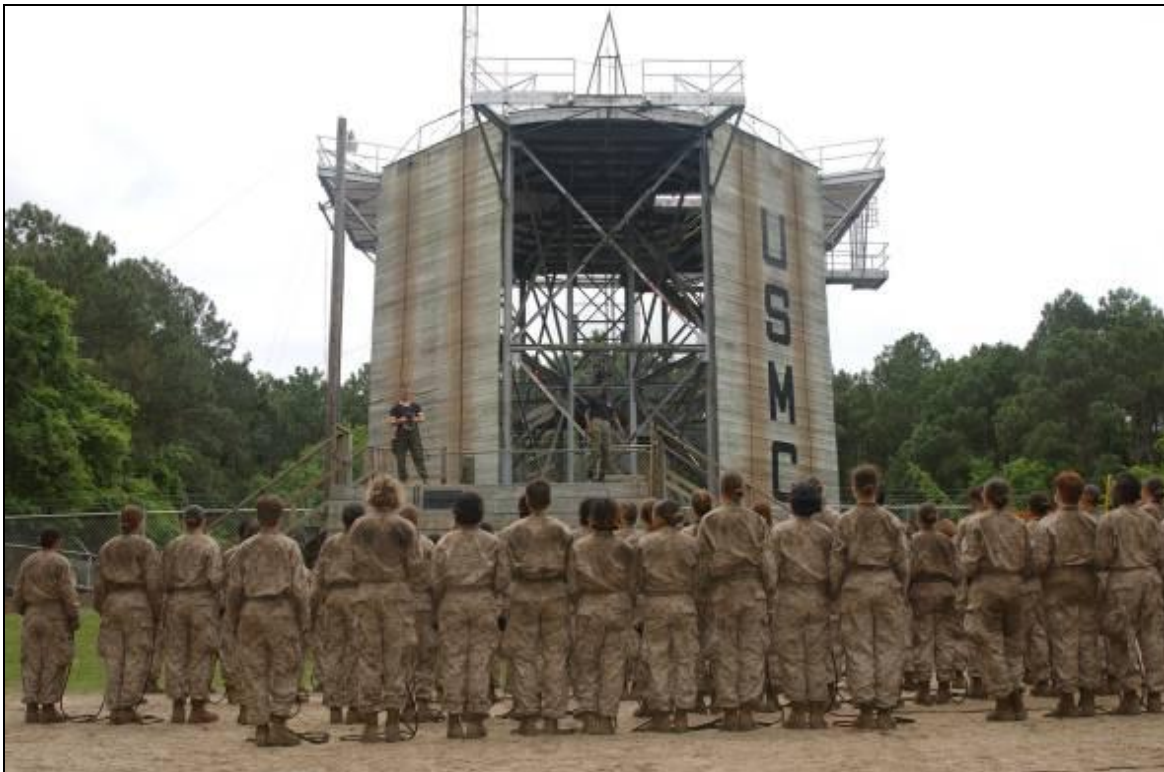
Figure 2.3-2. Example of Marine Corps Rappelling Tower
