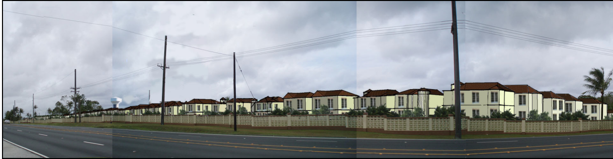
Figure 13.2-15. Alternative 3: View from Route 3 Looking Westward into the South Part of NCTS with Water Tower/Tank in the Background (RESULTING VIEW)
