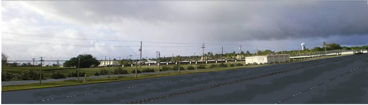
Figure 13.2-13. Alternative 3: Panoramic View from Route 3 Looking Northwestward into the Central Part of NCTS with New Warehouse in the Foreground and Water Tower/Tank in the Background (RESULTING VIEW) Source: EDAW 2010.
